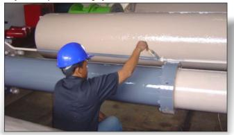
**CHEMCLAD® SC** - a two component, 100% solids, polymer system that creates an outstanding corrosion and chemical resistant protective coating on all types of equipment and structures.
