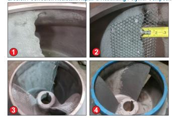
Outstanding erosion resistance. Trowelable system for repairing and rebuilding metal damaged by erosion and corrosion: on pumps, valves, heat exchangers, tube sheets, water boxes, etc.
