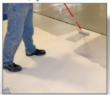
A two component, water-based, breathable coating system specifically designed to seal and protect concrete surfaces that may experience moisture problems. It resists blistering due to hydrostatic pressure and bonds to virtually any mineral / cement substrate as well as wood.
