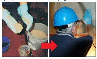
A cementitious, one component, extremely fast-setting product with the ability to stop running water through masonry structures. It is designed to be mixed with water and to set within one minute.
