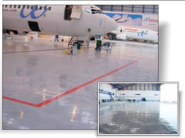
Easy to apply **ENECLAD**® seals and strengthens concrete floors. These high performance polymer composites are extremely abrasion resistant, making them ideal for heavy traffic areas in warehouses, hangars, loading docks, etc. They jacket the surface in a rugged coating that resists forklift traffic, oil, gasoline and most industrial chemicals.
