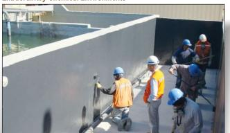
**CHEMCLAD® XC** is a two component, 100% solids, ultra high performance, chemical resistant coating that provides unrivaled protection in some of the toughest chemical environments.
