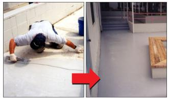
A three-component, 100% solids, concrete primer / sealer that is specifically formulated to smooth-out rough concrete surfaces in order to improve the appearance of ENECON® top-coats such as ENECLAD® FPS or CHEMCLAD®.
