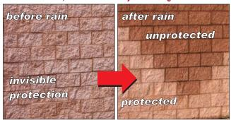
ENESEAL® MP is a single component, water-based, ultra-low viscosity weather barrier which dries to an invisible, water repellant masonry sealer. It provides extraordinary weather protection to virtually all types of concrete, masonry and mineral surfaces.
