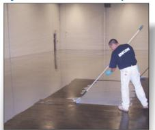
This extraordinary high performance polymer composite is extremely abrasion resistant, making it ideal for heavy traffic areas in warehouses, hangars, loading docks, etc.
