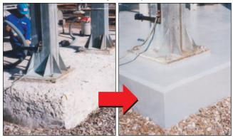
A three-component, 100% solids, concrete repair compound specifically formulated and precisely engineered to provide solutions to the most difficult concrete repair and protection problems. DuraQuartz LW is a light weight aggregate version for vertical and overhead surfaces.
